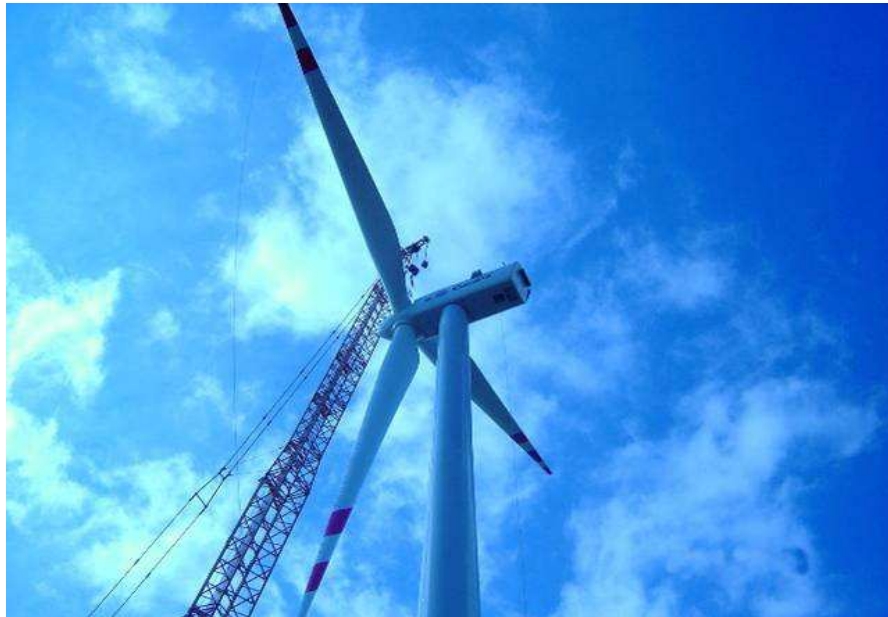
Assembling of Rotor
