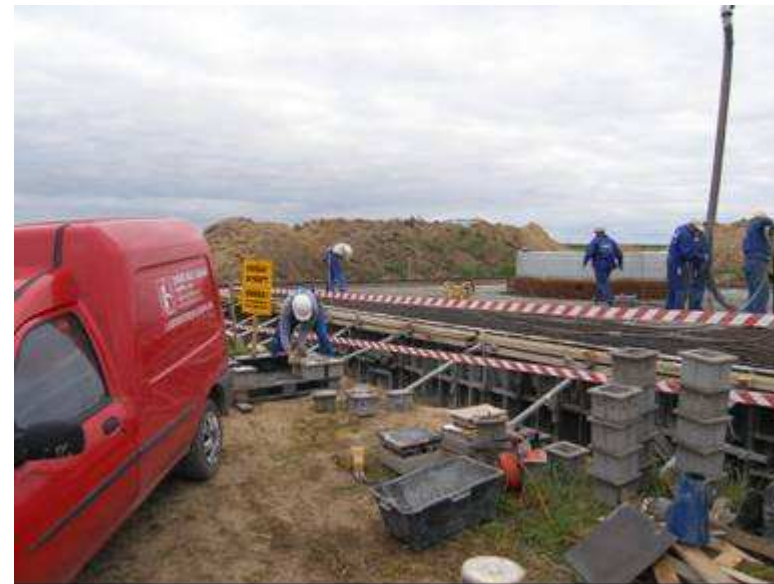
Laying concrete for the 8th turbine
